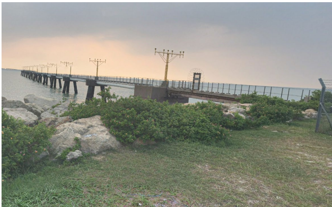
Figur 17: Innflygingslys, Hong kong International airport (bilde fra google)
